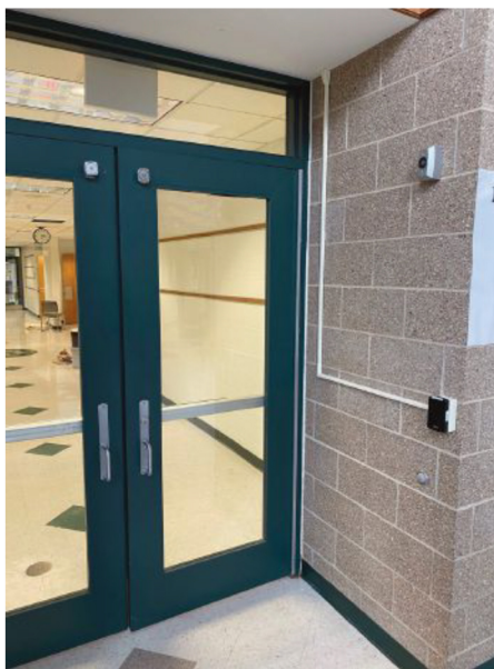
188 ISONAS RC-04 reader controllers were placed on every access point in the Chicago area school district's six buildings.
